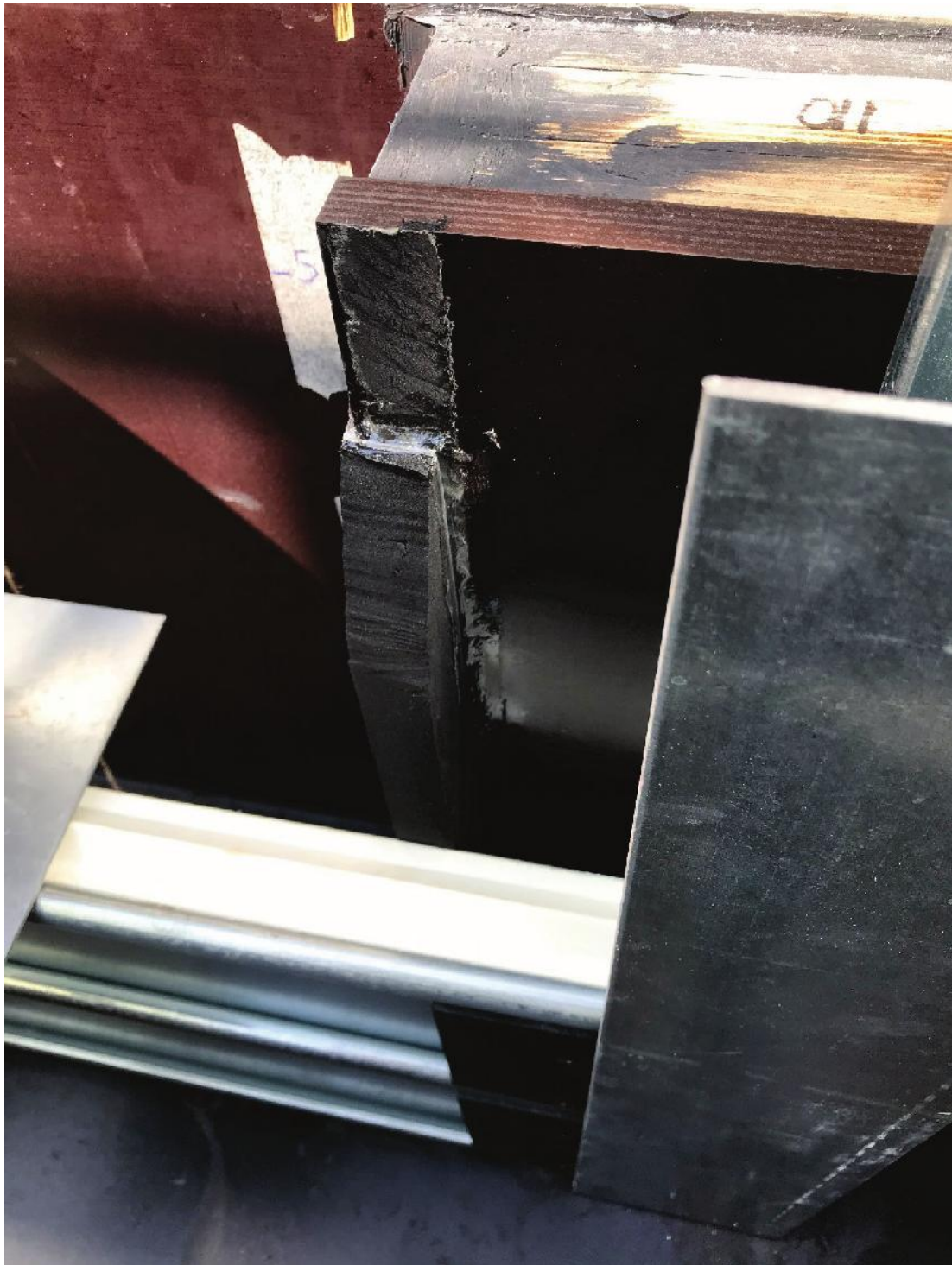
Photo B. 1.9 View of RGC seal, 300 mm test at the inside
